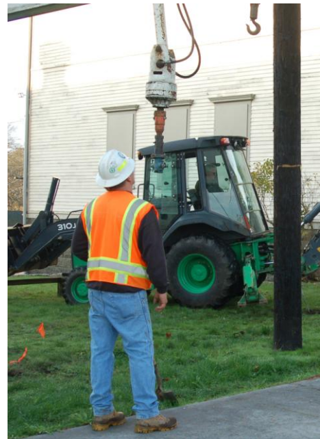
The line crew is lifting a load to the top of a pole
